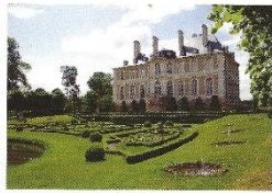
Château de Vendevier Gardens (Calvados) $10,000—New York Chapter Restoration project: The ornamental wrought-iron gate made in the first half of the 18th century that is in a perfect state. Built in 1741 on the place of Jacques François Blondel, the celebrated 18th-century architect, the château has been transmitted from father to son ever since and kept its original décor and part of its original furniture. It features important collections and notable gardens.
